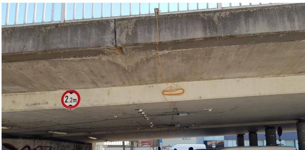
Fig. 1. Photo of the measuring sensors installed on the Vogelsang Bridge, Esslingen.
